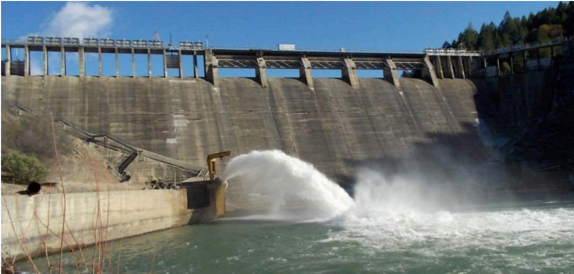
Scott Dam Spillway
