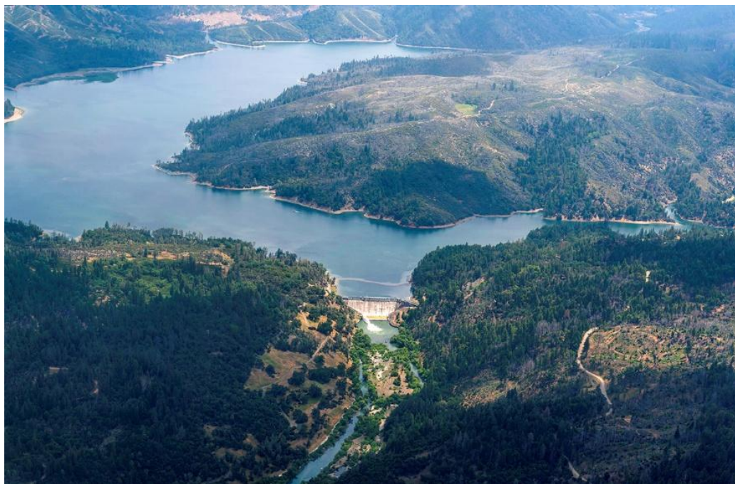
Scott Dam at Lake Pillsbury reservoir (photo: Friends of the Eel River)
